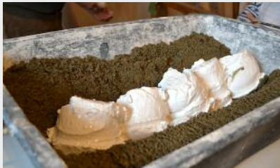
5. Lime mortar preparation: 2 parts inert (river sand)/1 part lime paste
