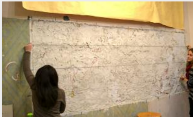
3. Preparatory drawing (Sinopia) on the arriccio, after dividing the space into a grid by "snapping the cords"
